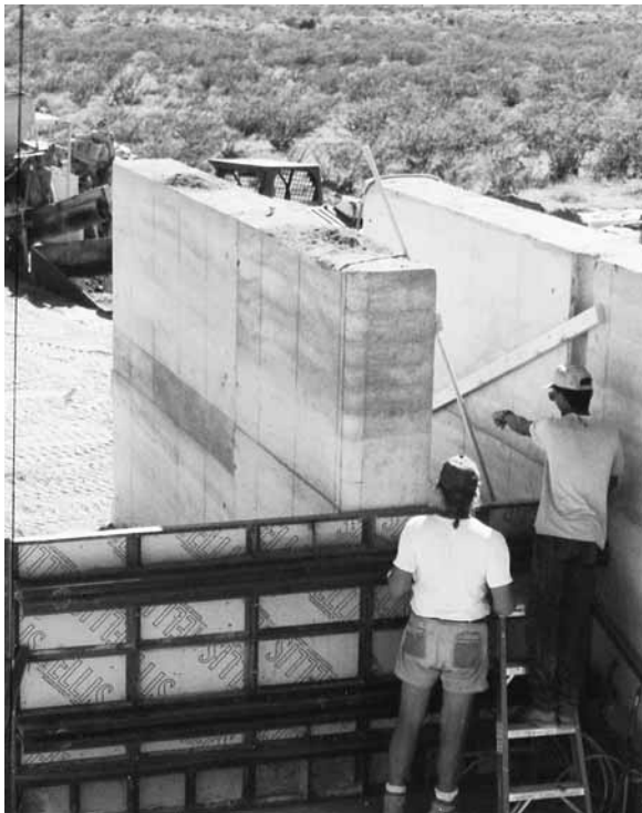
1.6: Rammed earth wall after removal of forms.
