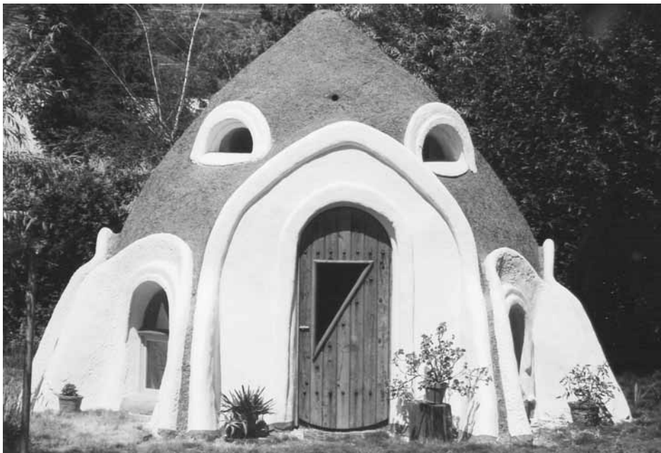
1.1: Using earthbags, a whole house, from foundation to walls to the roof, can be built using one construction medium.
