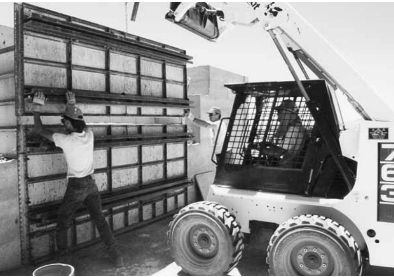
1.5: The entire form box can be set in place using the Bobcat. Steel whalers keep forms true and plumb and resist ramming pressure.
