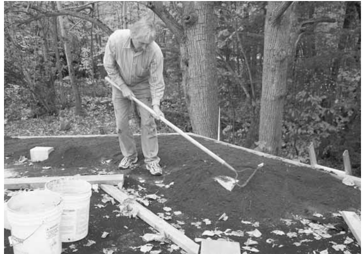
Fig. 8.11: The author uses the back of a rake to spread the soil to a consistent loose depth of 5½". Twenty-four 6-by-6-by-8-inch blocks (actually 5½" thick) served as depth gauges. The soil slumps down to the 3½" deep retaining timber. After a winter's snowload, the loose soil compressed to a compacted depth of about four inches.
