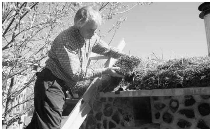
Fig. 8.16: The author installs a moss sod on the edge of the office roof.
