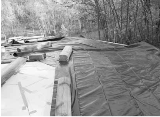
Fig. 8.5 (above): A layer of 6-mil black polyethylene serves as the base of the drainage layer and is installed over the insulation. This is tricky to do on an octagon roof, as the sheet needs to be folded over the saddles between facets, but it is an easy job on a Cave-type roof. We were careful to give plenty of overlap from sheet to sheet (at least 18") and paid attention to the shingle principal when making our overlaps.
