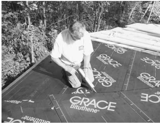
Fig. 8.2 (right): The author caulk the cut edge with Bituthene® Mastic.
