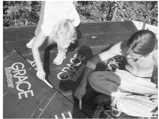
Fig. 8.3 (above): Jaki and Darin Roy feather the edge of the mastic with pointing knives, to approximate the factory edge of the Bituthene® membrane. The mastic stops the cut edge from raising up or "fish-mouthing."
