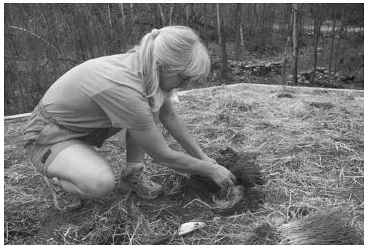
Fig. 8.13: Jaki plants a couple of dozen clumps of chives between 100 sedum plants (protected by mulch) on the Stoneview roof. Sedum is a succulent plant with the ability to survive prolonged drought conditions. Chives also do well in dry conditions.
