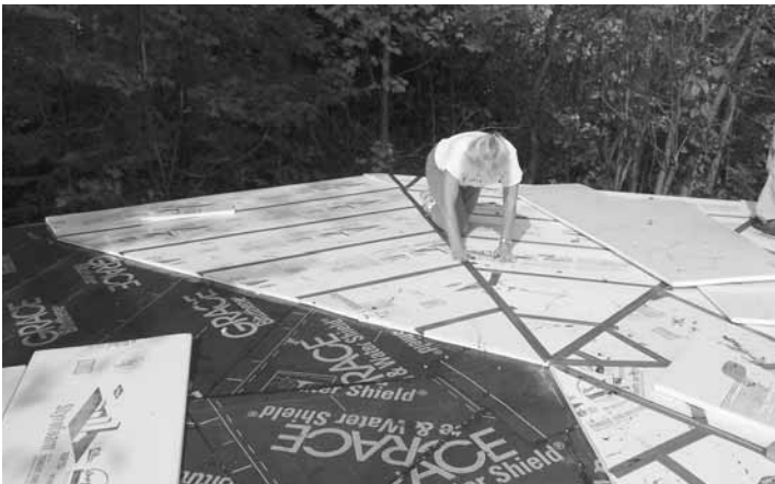
Fig. 8.2 (right): The author caulk the cut edge with Bituthene® Mastic.
