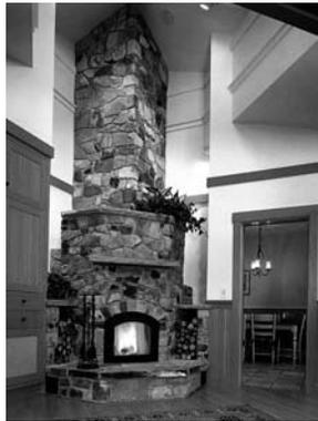
Temp-Cast is a modular masonry heater core kit featuring corner, 'see through,' and bake-oven models. Temp-Cast provides manuals detailing appropriate chimney construction with each masonry heater kit. Masonry materials for the chimney and the heater's exterior are sourced separately.
