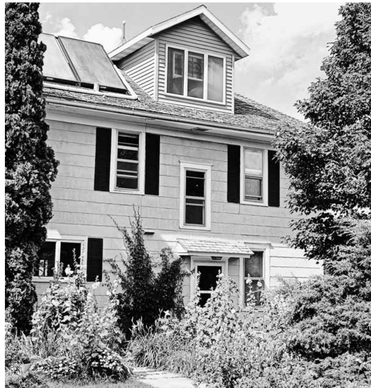
Inn Serendipity farmhouse with solar thermal system on roof, used to heat domestic hot water.
