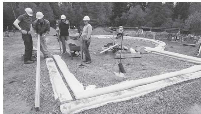
Earthbag foundation. (DAVID ELFSTROM)
