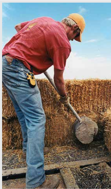
FIGURE I.2. Natural building emphasizes the use of inexpensive tools and simple, easy-to-learn techniques. Here, a mallet fashioned from a log is being used to tap straw bales into place. This building was the first straw bale demonstration project organized by the American Indian Housing Initiative at the Crow Indian Reservation in Montana in 1999. [Credit: Michael Rosenberg]
