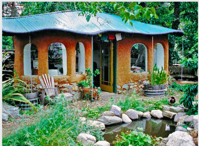
FIGURE 1.3. At the Permaculture Institute of Northern California, designers pride themselves on “closing loops”—filling needs with local resources while minimizing waste and environmental impacts. For example, the clay for this cob and straw-clay hybrid office was dug from a hole (right front) that later served as a duck pond and part of the site’s greywater recycling and rainwater collection system. [Credit: Michael G. Smith]
