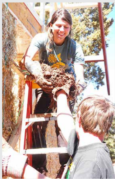
FIGURE 1.4. Natural building techniques allow people with minimal training to work together to build an inexpensive home. These systems often require a lot of labor but little cost in materials and tools. Here, workshop participants apply a base coat of clay plaster to a straw bale wall. [Credit: Catherine Wanek]
