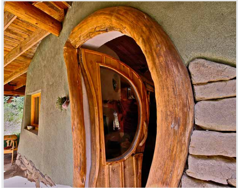
FIGURE 1.6. Come on in—the door is open! This family home in British Columbia, built by Cobworks in collaboration with the homeowners, combines cob walls, local stone foundations, milled and unmilled wood and natural plasters. [Credit: Misha Rauchwerger]
