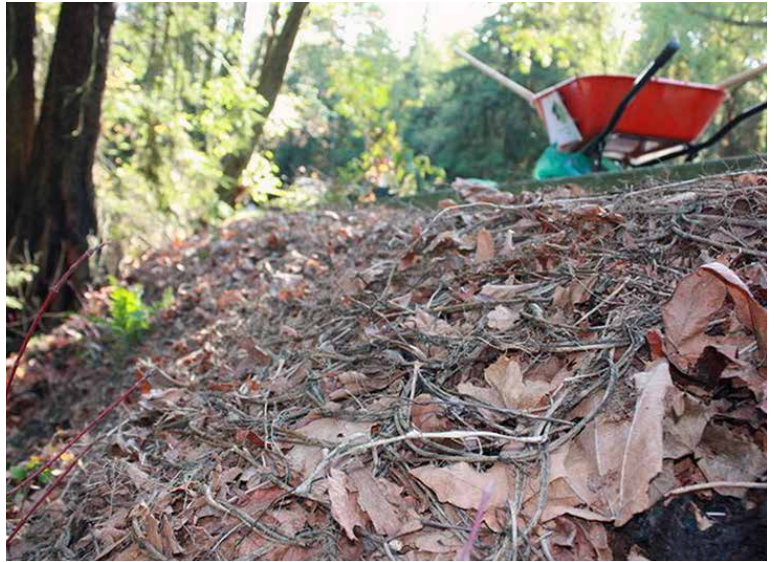
Fig. 1.10: Ivy netting installation complete.
