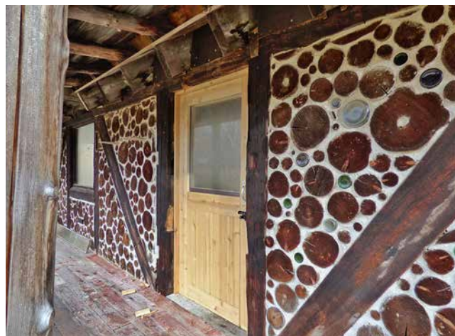
1.13. Log End Cottage, built in 1975. Doors and windows are enclosed by the timber frame itself, mostly 8-inch by 8-inch recycled barn beams.
