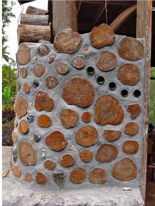
1.20. Exterior view of a "mini" bull-nose corner, wrapping around an ohia post in a timber-framed home in Hawaii. Small log-ends and chunks of lava helped fill large mortar joints.
