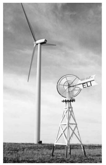
**FIGURE 1.1.** Water-pumping windmills like this one, photographed by Dan on a commercial wind farm in southeastern Colorado, were once common through the West and Midwest. The technology is so good that it hasn't changed in 100 years. Credit: Dan Chiras.
