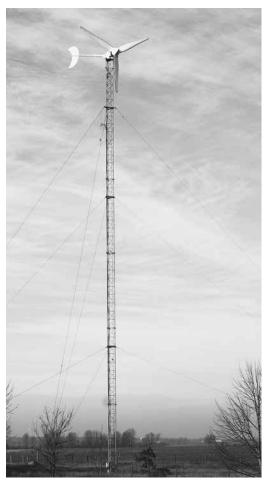
FIGURE 1.4. Small Wind Turbine on Tower. This ARE442 wind turbine installed at Mick's house during a workshop is mounted on a guyed lattice tower. Maintenance is performed by climbing the tower. The ARE442 is now manufactured and sold by a company called Xzeres. The turbine is called the Xzeres 442SR. Credit: Dan Chiras.
