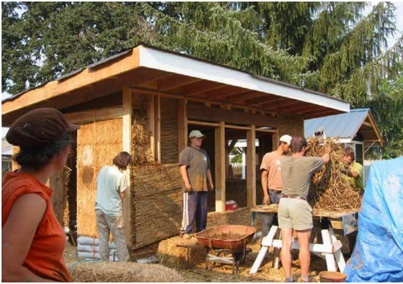
Straw bales are load bearing in this building that uses LSC for the south wall.
