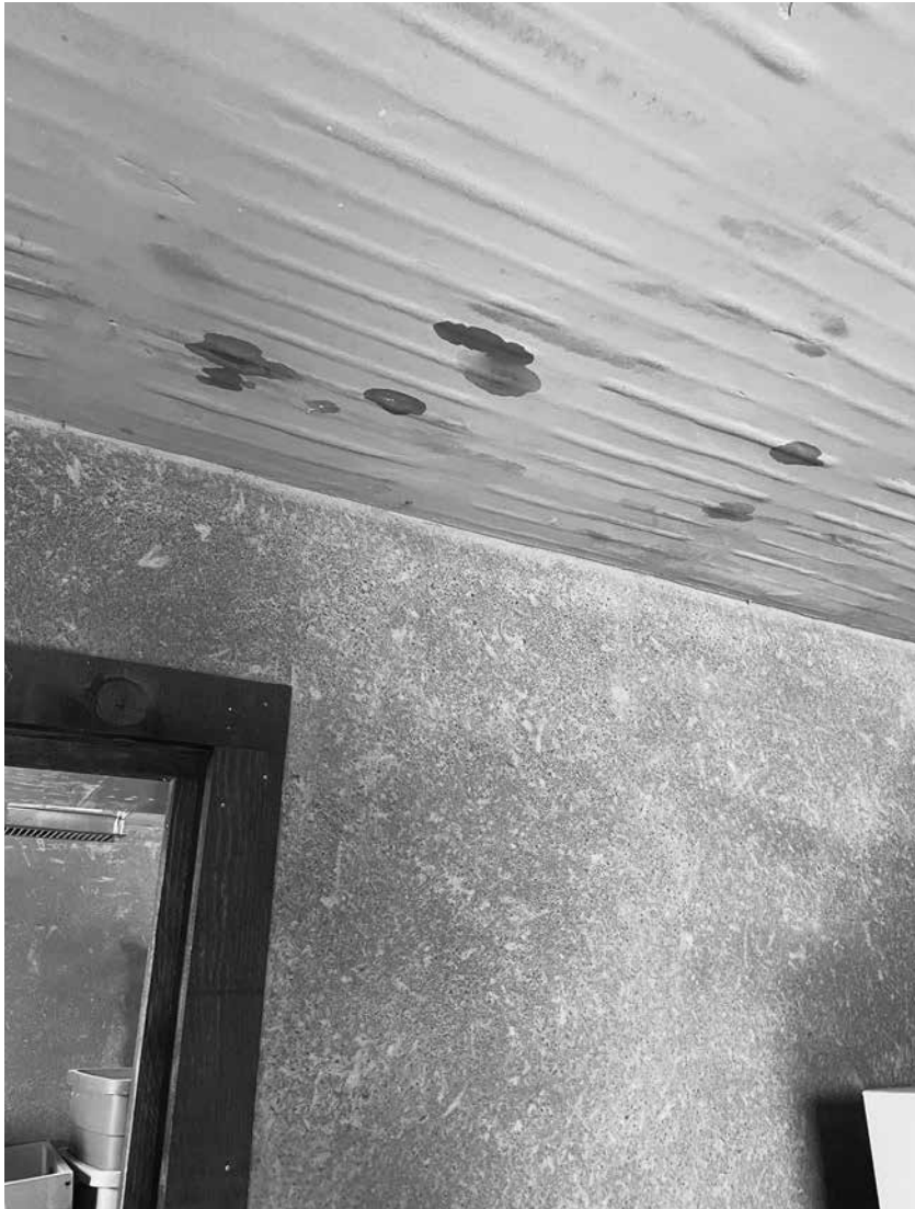
Fig. 1.6: Water is starting to find a way through this green roof after 10 years.
